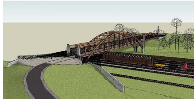
A bike / pedestrian bridge will be built to span active rail yards and connect Mitchell Park to the Valley.
