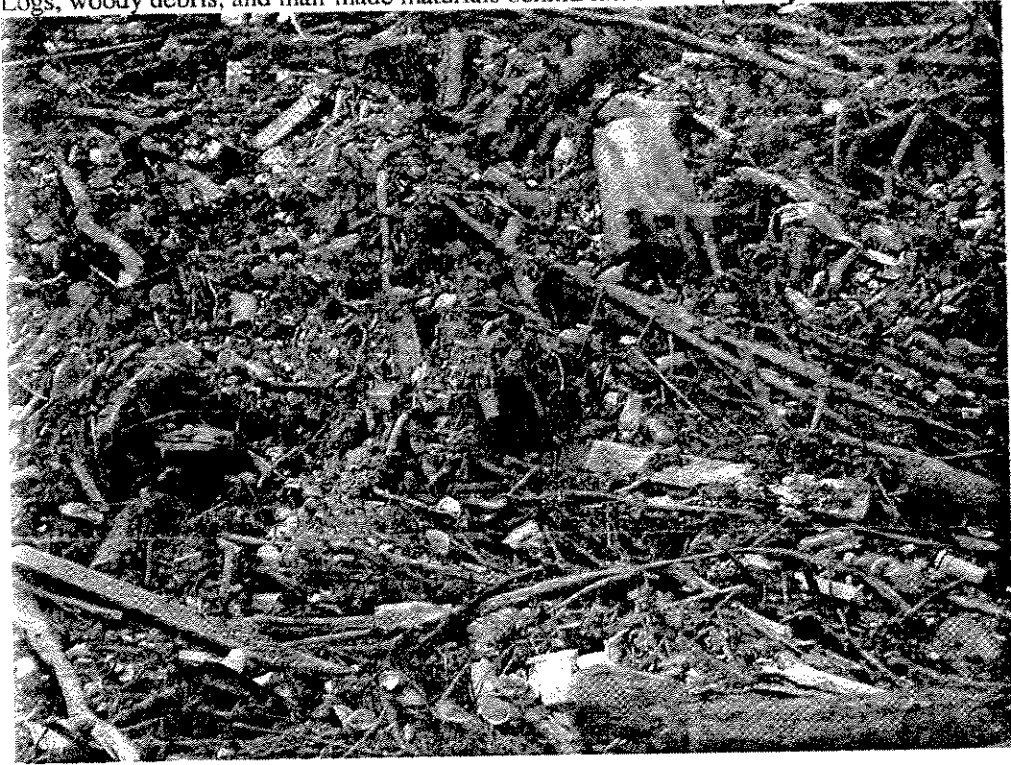
Logs, woody debris, and man-made materials behind fixed crest spillway (November 17, 2000):
