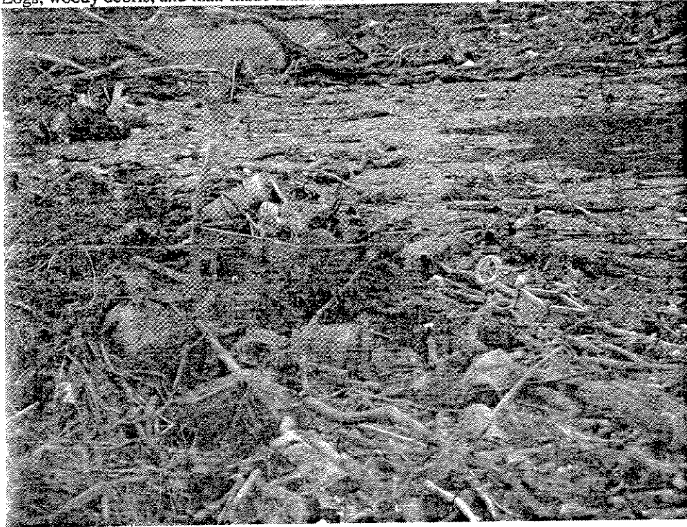
Logs, woody debris, and man-made materials behind fixed crest spillway (October 27, 2004):
